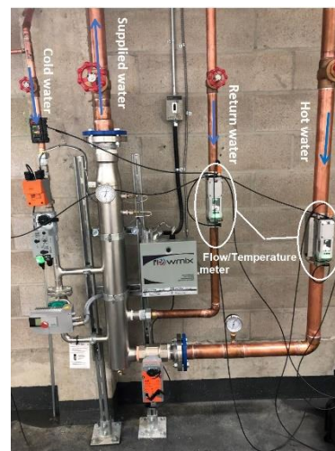
b) DHW system with the Flowmix
